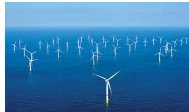
We've come a long way from old-fashioned windmills. Wind energy turns the blades of a turbine, which feeds an electric generator and produces electricity. Wind, which accounts for 9.2 percent of US electricity generation, has become one of the cheapest sources of energy in the country. The top states for wind power include California, Iowa, Kansas, Oklahoma and Texas, although turbines can be placed anywhere with high wind speeds - such as hilltops and open plains.
